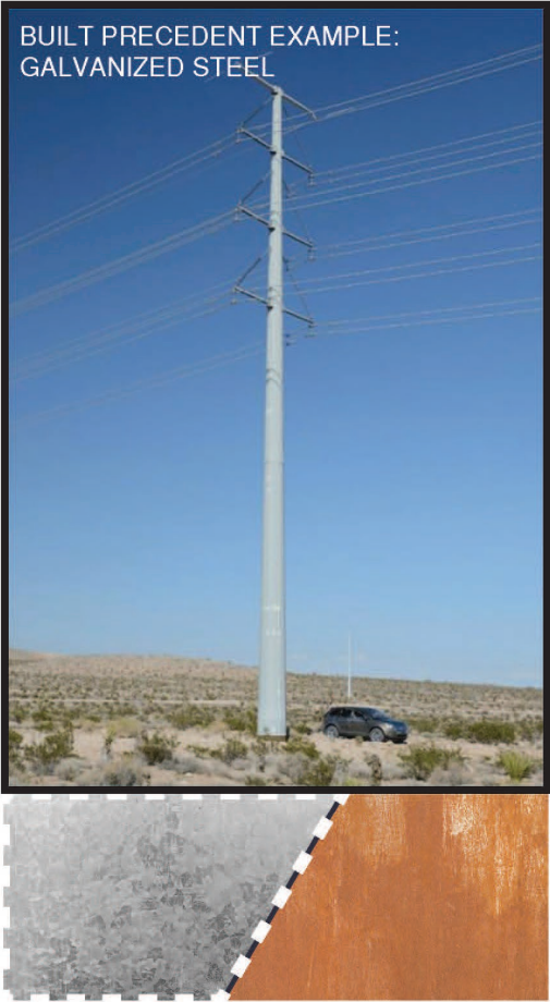
Representative Monopole Building Material Comparison: Galvanized Steel vs Weathering Steel Finish
